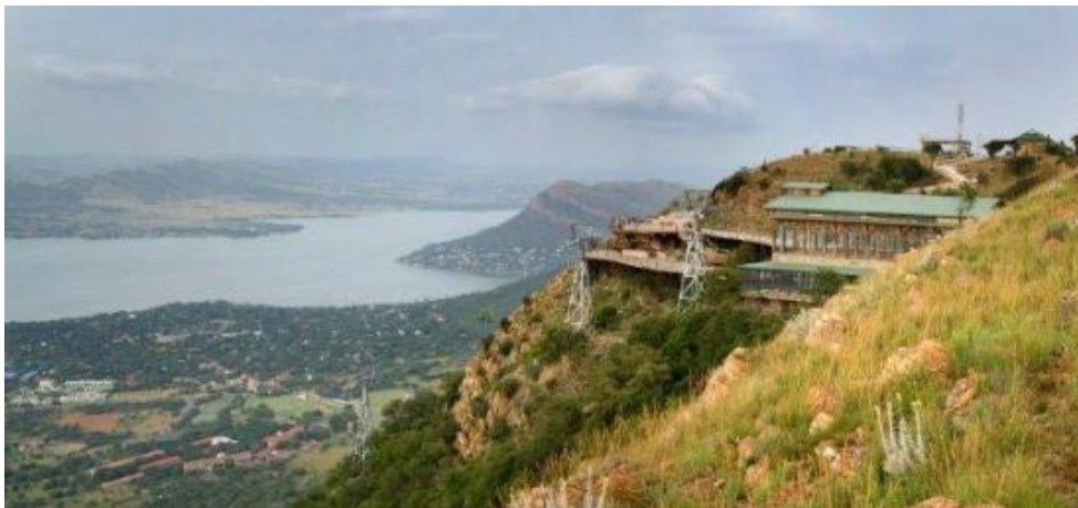
Picture: The Upper Station of the Hartbeespoort Cableway
